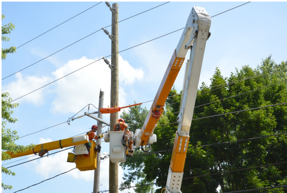
Alectra's Line maintainer's working on rebuilding overhead infrastructure.
